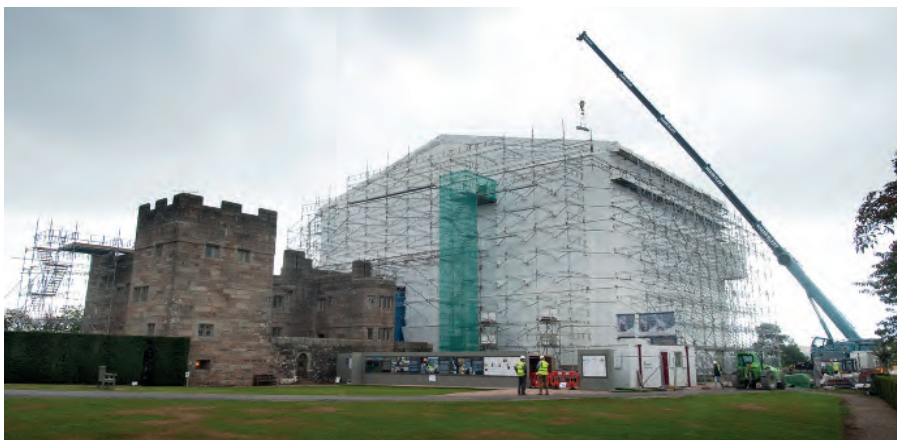
The 100-tonne crane (above) used at Drogo to lift the lintels before they were carefully positioned over the windows (below). © Stephen Hayward
